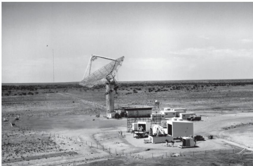
Fig. 17.6. Radar at Central Bore near Mt. Elba at Woomera. This Stanford Research Institute-built radar and the optical site in the foreground were established in 1964–1965 for the *Dazzle* program studying plasma trails in the wakes of reentering bodies. Communications, tracking, and instrumentation sites spanned a huge territory claimed by the Woomera test range and its remote impact areas. Photo courtesy of Defense Science and Technology Organization, Department of Defense, Australia.
