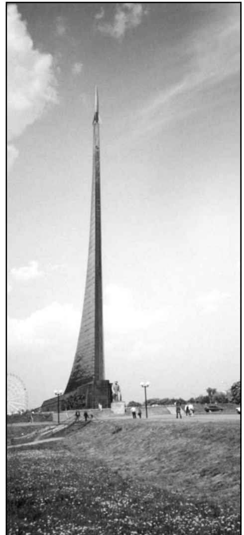
Figure 1. Monument to the conquerors of space opened in Moscow in 1964 (photo taken in 2001). The upper 99-m (325-ft) part of the monument is made of titanium and steel; the rocket on the top is 11 m (36 ft) tall.
