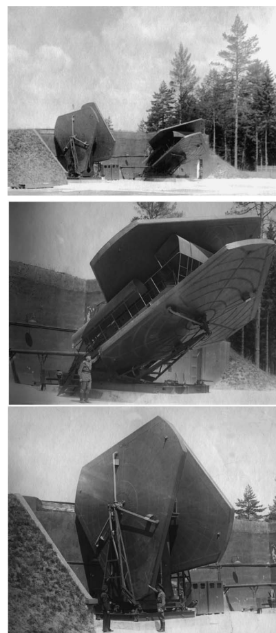
Fig. 1. Track-while-scan B-200 (Yo-Yo) radar (top) with heights of the azimuth (middle) and elevation (bottom) units 8 and 9 m, respectively. Photographs from [5].
