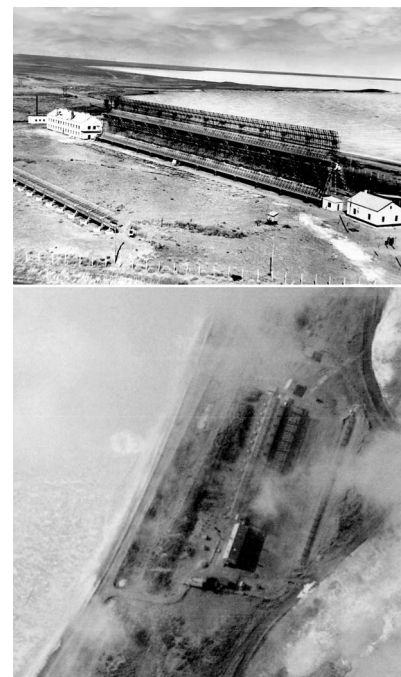
Fig. 5. Receiving antenna of the long-range Dunai-2 (“Hen Roost”) radar on the shore of Lake Balkhash. Top: photograph [9] courtesy of Mikhail Khodarenok; bottom: original photograph (U-2 Mission 4155; April 9, 1960) from National Archives and Records Administration; photograph identification, interpretation, and processing by Mike Gruntman.
