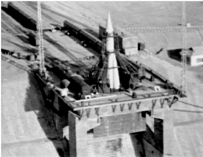
Fig. 8. R-7 ICBM readied for launch at Tyuratam in May–June 1957. The platform stands out as a cliff over the gigantic flame pit beneath. The first ICBM, first artificial satellite, and first cosmonaut were launched from this technical position, Site 1. The installation is operational until this day, sending Soyuz launchers to space. Photo courtesy of Videocosmos. From Ref. [56].
